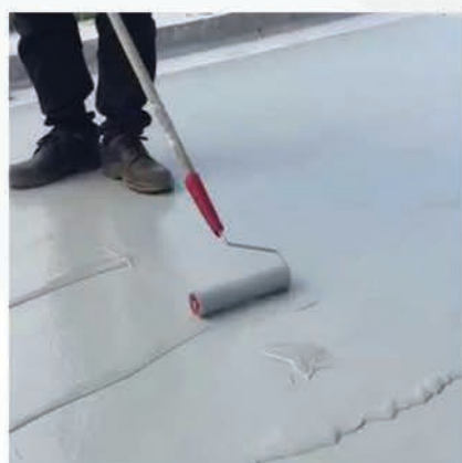
Chemical Waterproofing
