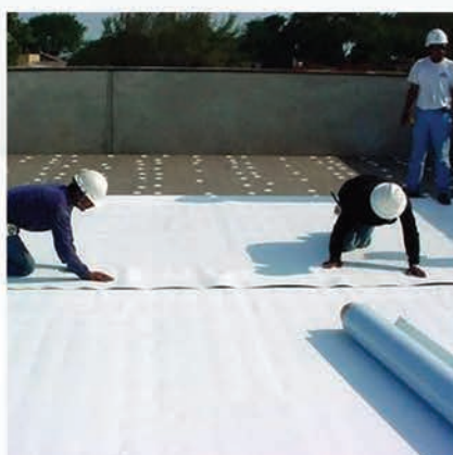
PVC Membrane Waterproofing
