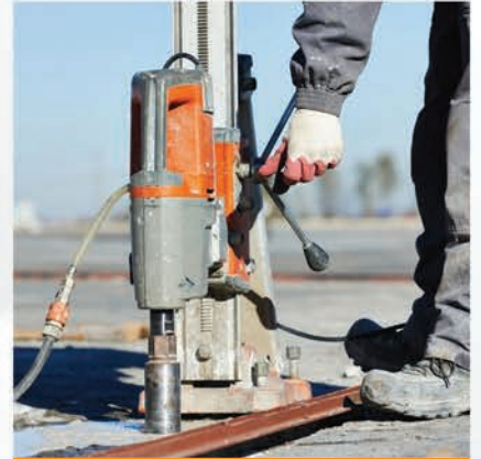
Concrete Coring
