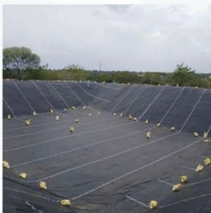
HDPE Membrane Waterproofing
